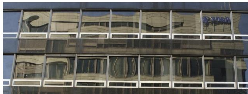
Figure 1. Real-world glass reflection. Notice that reflection in different windows on the same facade can appear very different due to minor deformations and normal variations. Our goal is to capture normal maps of real windows to faithfully reproduce this effect.
